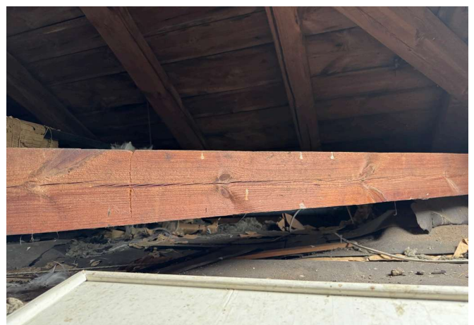
037c Seevilla, Dach
